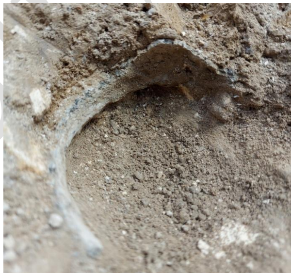
Figure 10 – Possible Lead Pipe Join
